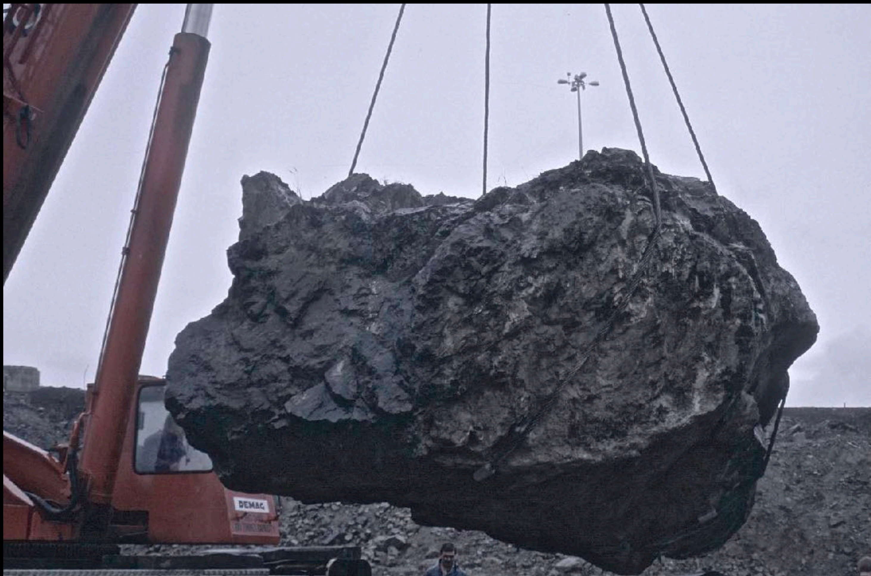
Lifting with 200 ton crane
